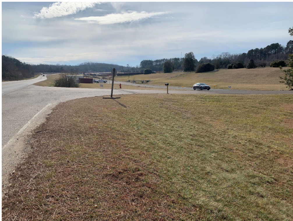
Industrial Driveway Crossing
