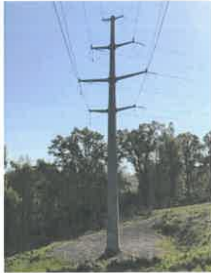
FIGURE 2 REPRESENTATIVE PROPOSED DOUBLE-CIRCUIT, SINGLE POLE STRUCTURE
