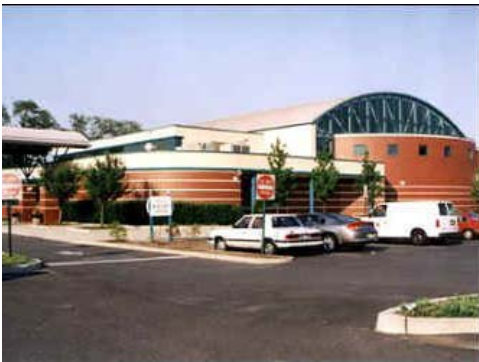
Indoor Recreation Center.
